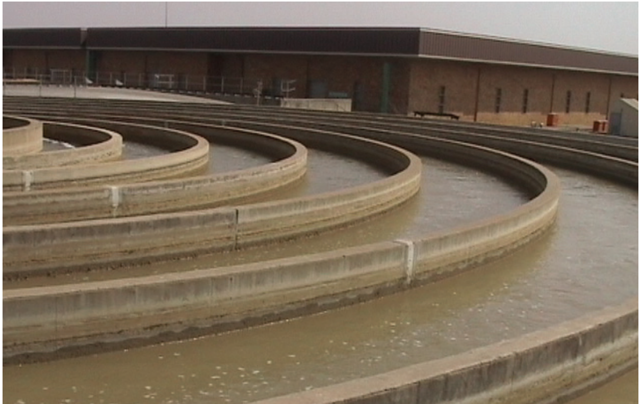
Figure B1.6: Spiral flocculator
