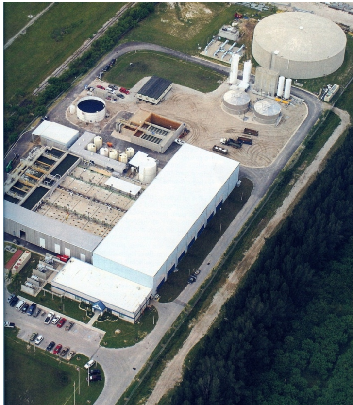
Figure 4: Layout of the Tampa Bay SWRO Desalination Plant, Florida
