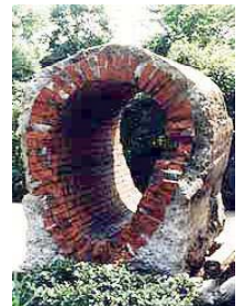
Fig. 3.2 Japan's first modern sewerage built in Yokohama 1881-1883
