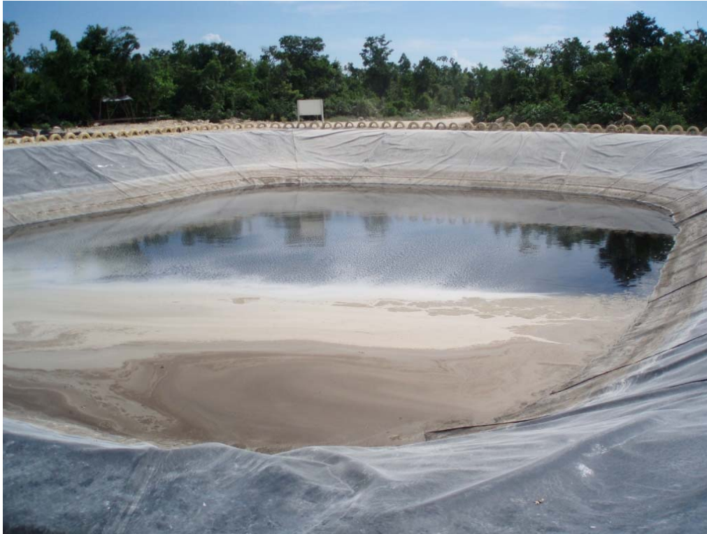
Figure 11 – Geo-membrane Evaporation Pond Liner
