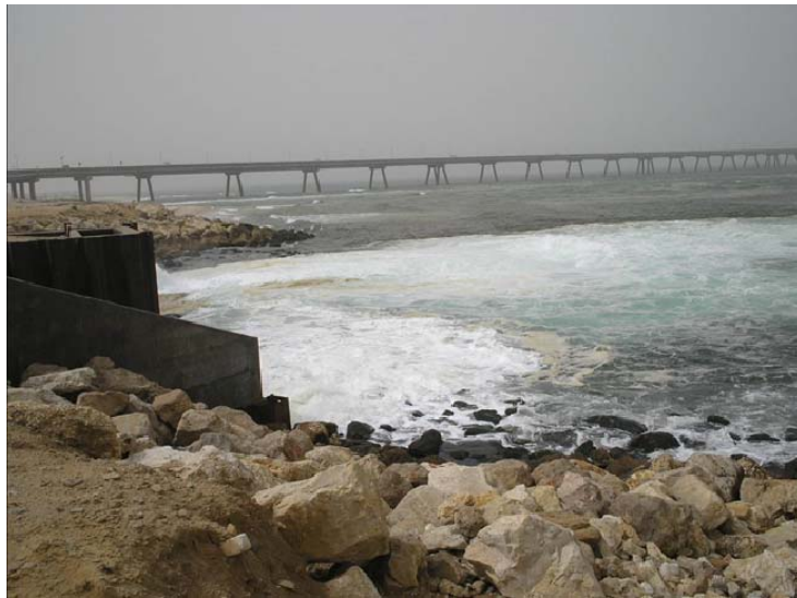
Figure 5 – 85 MGD Ashkelon Desalination Plant Near-shore Discharge
