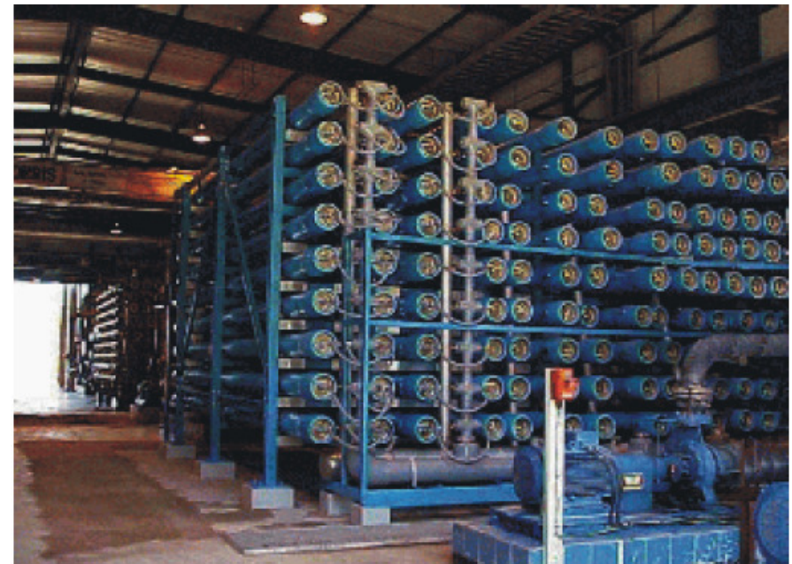
The Umm Lujj Nanofiltration Plant for Pretreatment of Seawater Before Reverse Osmosis
