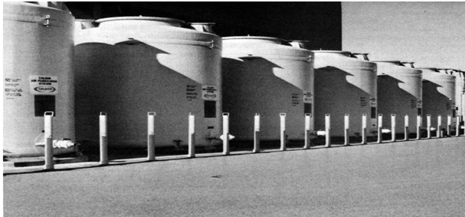
Figure 1.6 A large-scale activated carbon system 10
