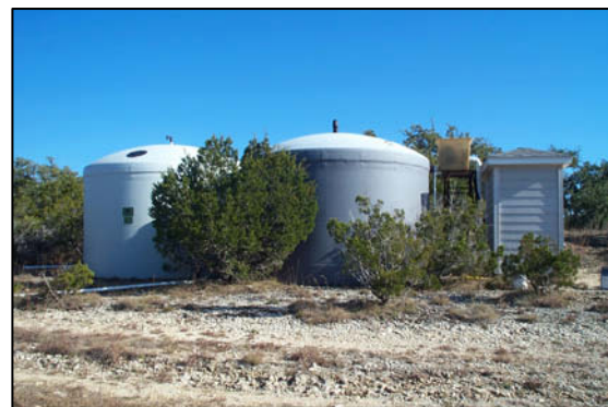
Figure 2-5. Two 10,000-gallon fiberglass tanks
