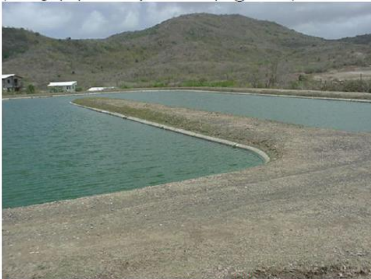
Aerobic Lagoons, St. Lucia (Courtesy CEHI)
