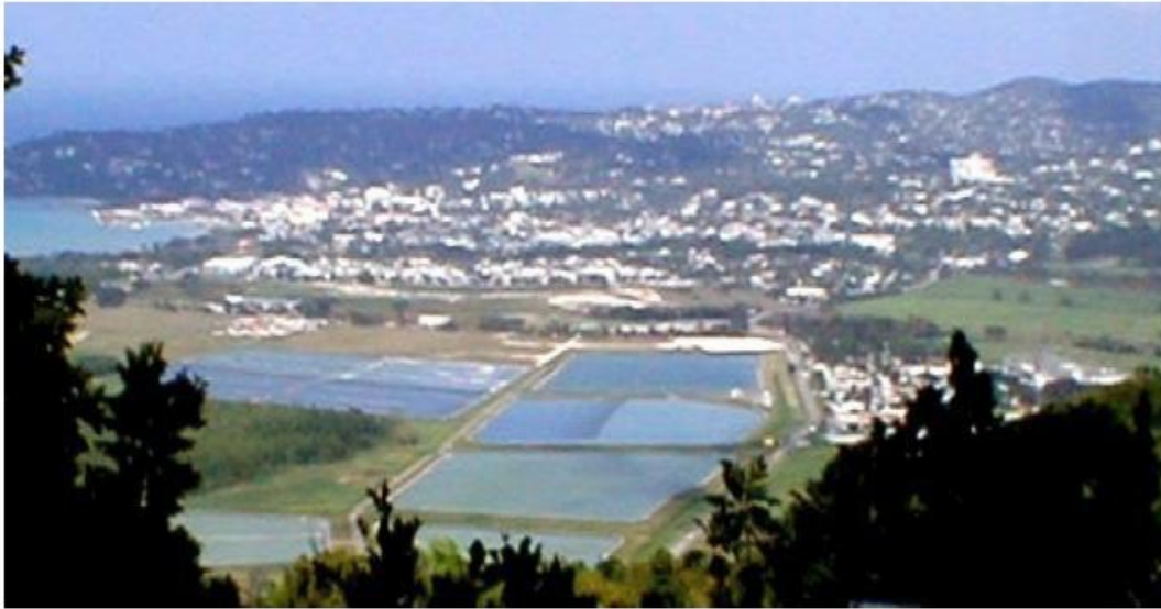
Facultative and maturation ponds in series for treatment of municipal wastewater in a city in Jamaica. (Photograph provided by UCYConcepts@aol.com)
