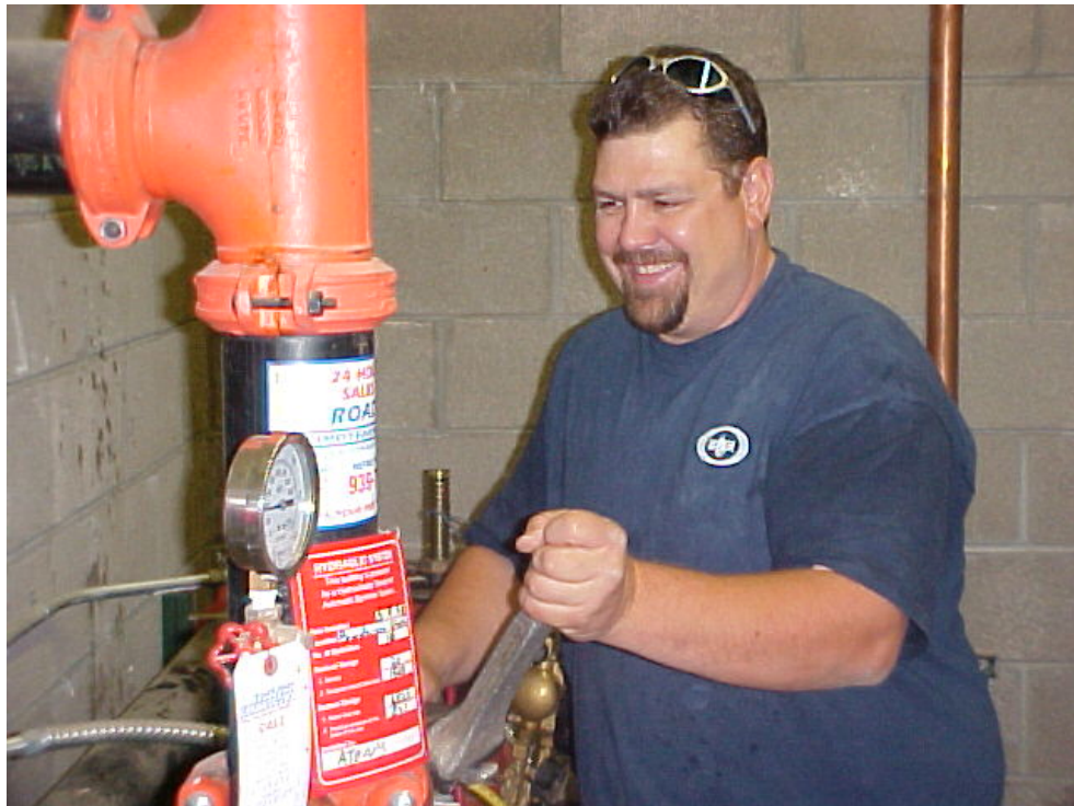
Top, a highly trained General Backflow Assembly Tester is working on a fireline assembly. Bottom, a double check backflow preventor with OS& Y valves.
