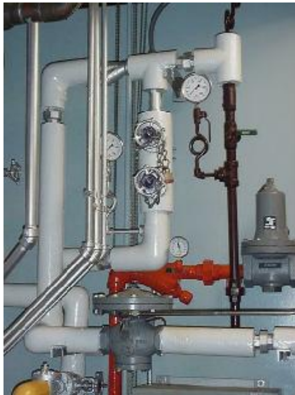
Notice the chain for locking the wheel valve.
