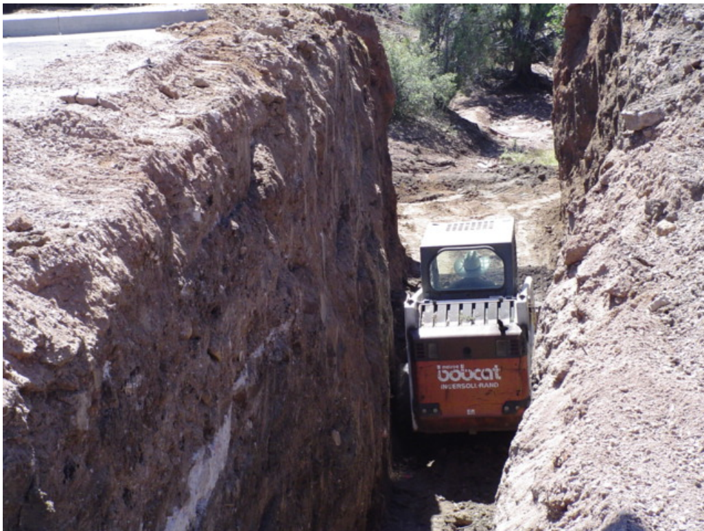
Major OSHA Violation. Do not operate equipment in unprotected trenches. This guy is trying hard to get to Heaven before his time is up.
