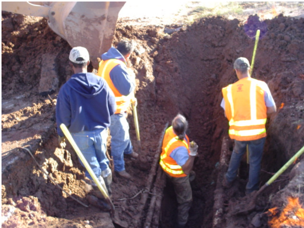
Two unsafe excavation examples: Top, notice the man in a 6 foot deep trench with no ladder or shoring, and the placement of spoil. Bottom picture, utilities are marked after the excavation has begun, no hard hats, no ladders, no protective system, incorrect spoil placement.
