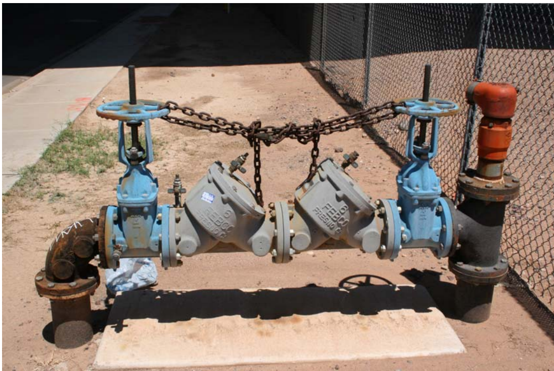
Top, a highly trained General Backflow Assembly Tester is working on a fireline assembly. Bottom, a double check backflow preventor with OS& Y valves.
