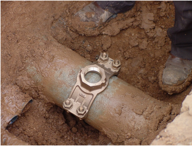
Installation of a new customer water service line.
