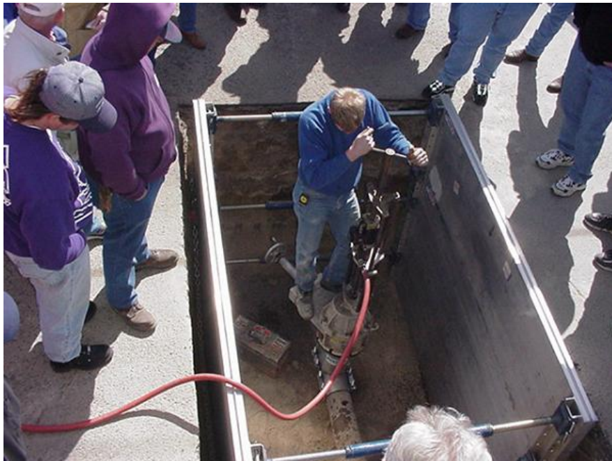
Hydro-Stop valve insertion machine
