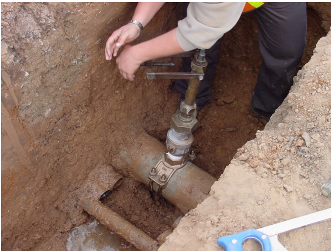
Installation of a new customer water service line.
