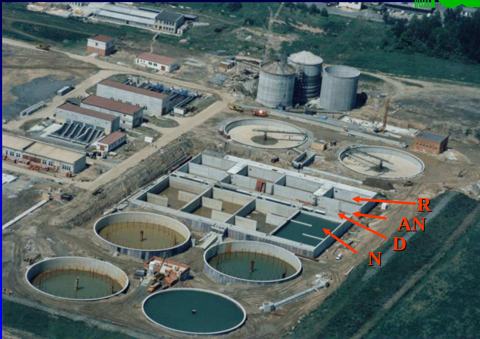
Pilsen WWTP under construction
