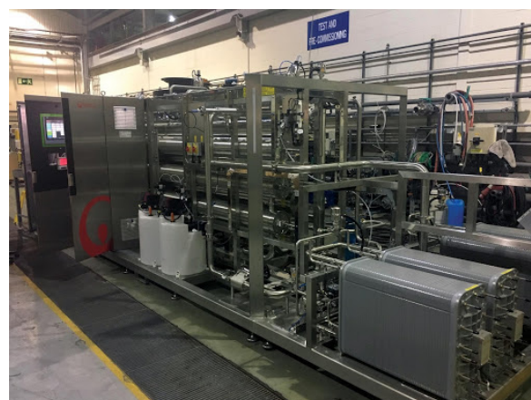
Test of ORION in UK
