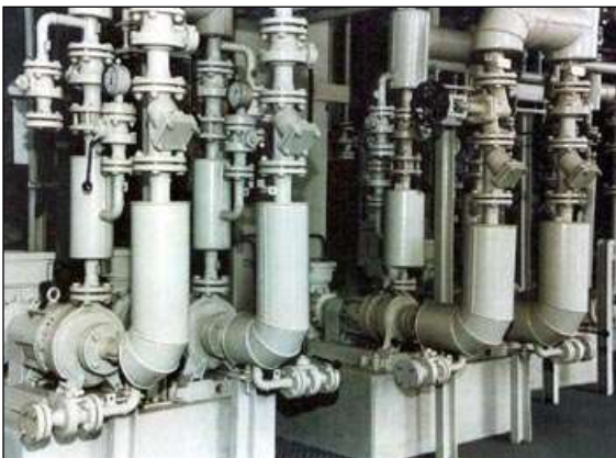
Magnetic drive centrifugal pumps with metallic containment shells
