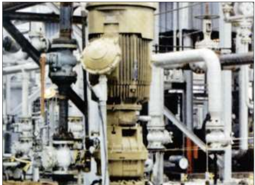
Photo 1. A centrifugal pump performing high speed/low flow duties in a Gulf Coast plant.
