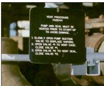
Photo 2. Seal and pump venting procedure
