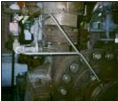
Photo 1. Piping reinforcement detail
