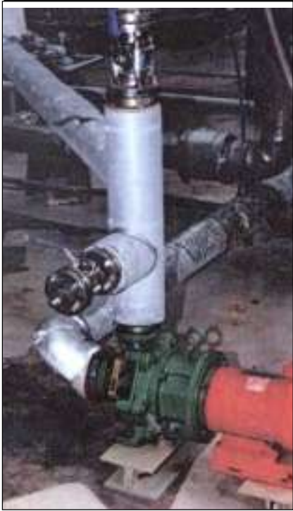
Photo 2. A mag drive pump transferring 50% sodium hydroxide at a specialty chemical manufacturer in the southeastern U.S.
