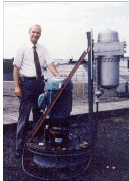
Photo 1. By slurring the scum blanket with a recirculating chopper pump, Tony Kucikas of Nut Island WWTP rejuvenated the digester and saved Boston $1.5 million in cleanout costs.
