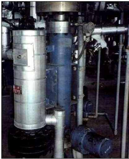
Photo 3. This canned motor-under pump at a chemical processing facility – an end suction configuration – has to contend with entrained gas and thermal shock.
