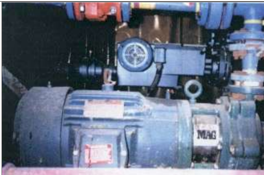
Photo 1. Mag drive pump transfer of 93% sulfuric acid has operated nearly two years without repair
