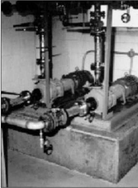
Photo 3. Upgraded pump site includes epoxy base and grout for improved reliability.
