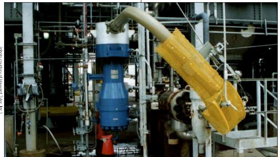
Photo 2. A 6000 psig/300°F canned motor-under pump in service at a chemical process plant. Large quantities of gas are injected and consumed as part of the process. This gas becomes entrained and the primary concern is loss of liquid in the pump end. The process has upset conditions with rapid pressure spikes to 6000 psig .
