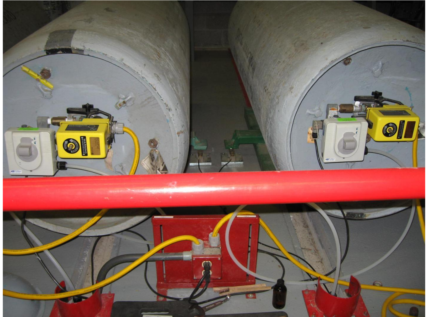
1-ton chlorine gas cylinders
