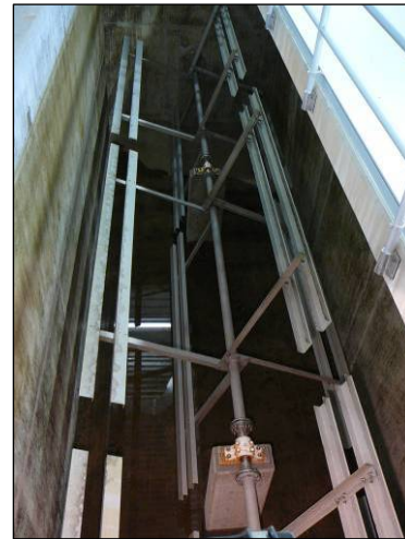
Figure 14: Flocculator designs Maze Flocculation Basin Left, Rotating horizontal Pickets (paddles) Right. Photos by author.
