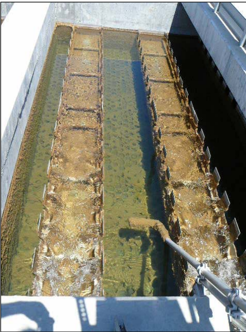
Figure 32: Tube Settlers enhance settling
