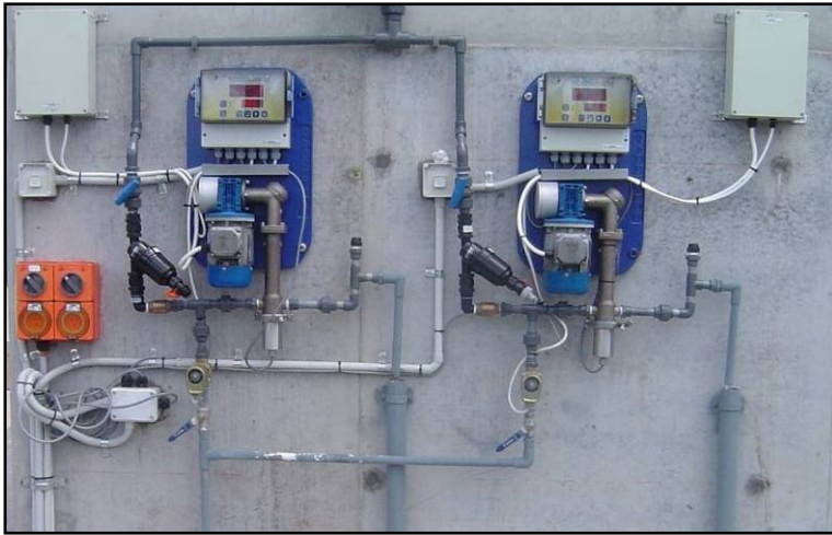
Figure 24: Accufloc Streaming Current Monitor. Photo used with permission of Accurate Measurement, LTD.
