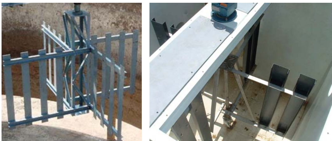
Figure 7 Flocculation stirring paddles.
