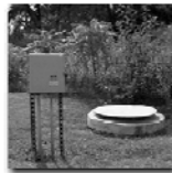
Submersible (S) stations are designed to direct traffic with colored markings, used there to group hoses and there is a network of alarm ground equipment. Drains to lower ground conditions are more and less safety hazard concerns.
