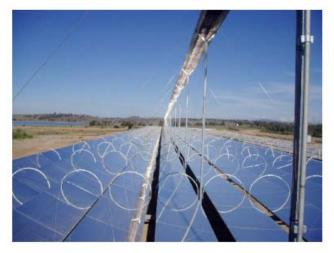
Figure 7: Linear Fresnel collector (Ausra)
