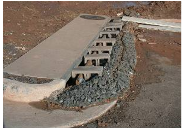
Coarse gravel and cinder blocks are often used to keep sediment and other pollutants out of storm drains
