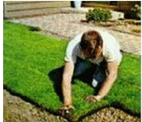
Grass sod is laid on exposed soil to stabilize the soil and to reduce the velocity of storm water runoff (Source: Landscape USA, no date)
