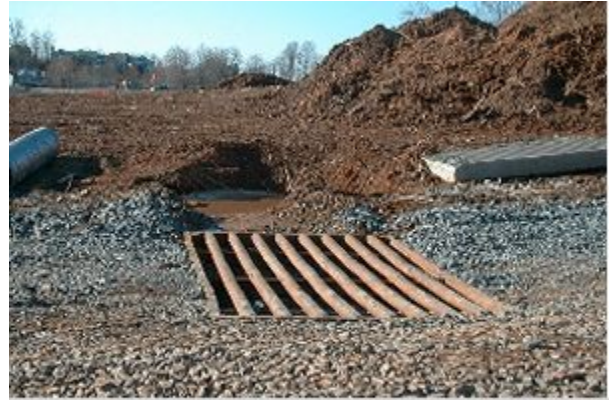
Stabilized construction entrances allow dirt to be removed from tire treads and collected as trucks leave construction sites
