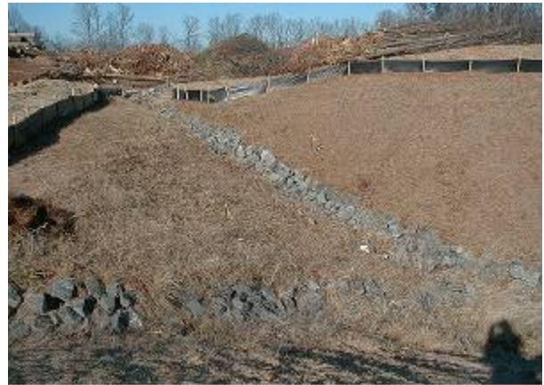
Riprap can be used to stabilize drainageways and outlets to prevent erosion
