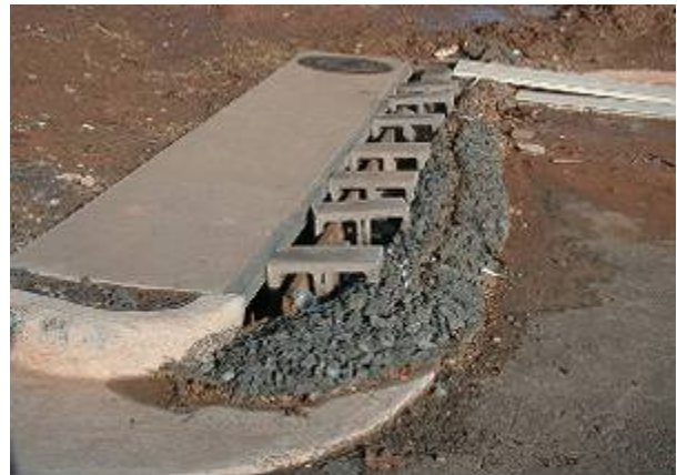
Coarse gravel and cinder blocks are often used to keep sediment and other pollutants out of storm drains
