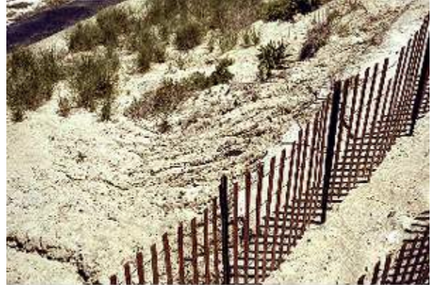
Sand fences are used to trap blowing sand and to reduce offsite movement of sand particles
