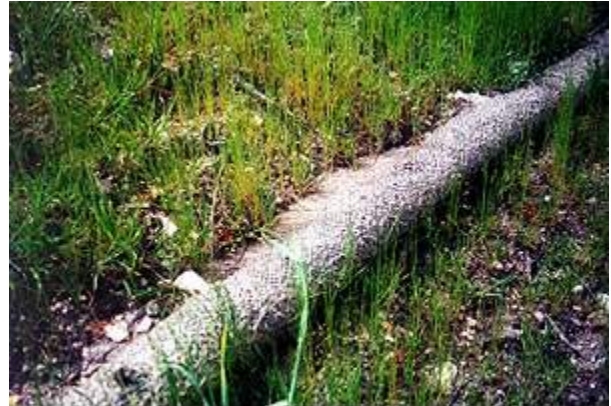
Brush barriers trap sediment and remove pollutants from storm water
