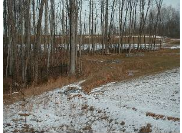
Diversion dikes can be used to contain storm water onsite
