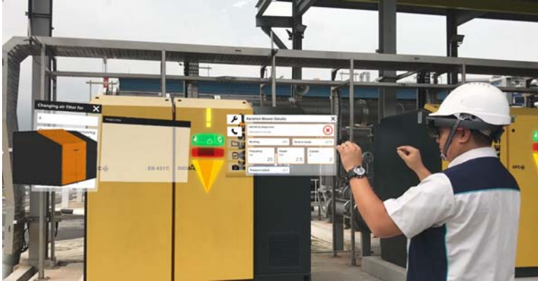
Figure 3.11 Use of AR to support on-site maintenance work.
