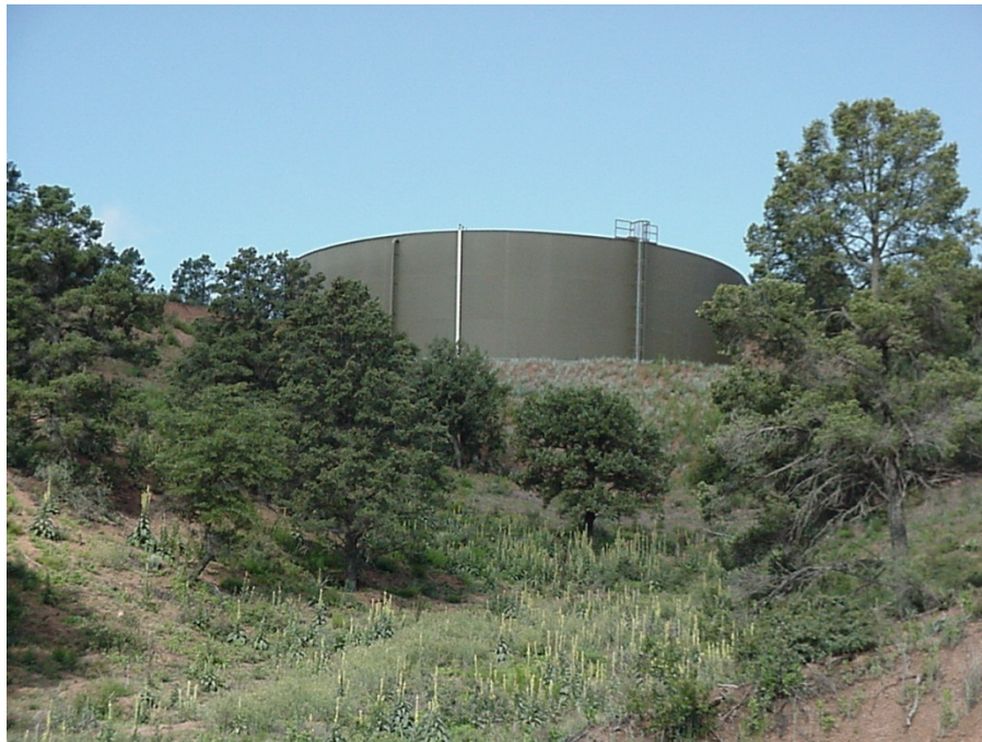
Large steel water storage tank
