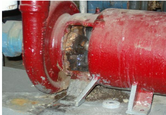
Figure 2.1 Leaking Gland
