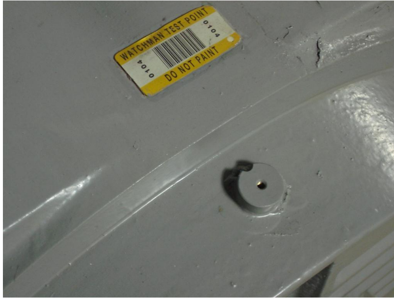
Figure 2.2 Vibration Analysis Point
