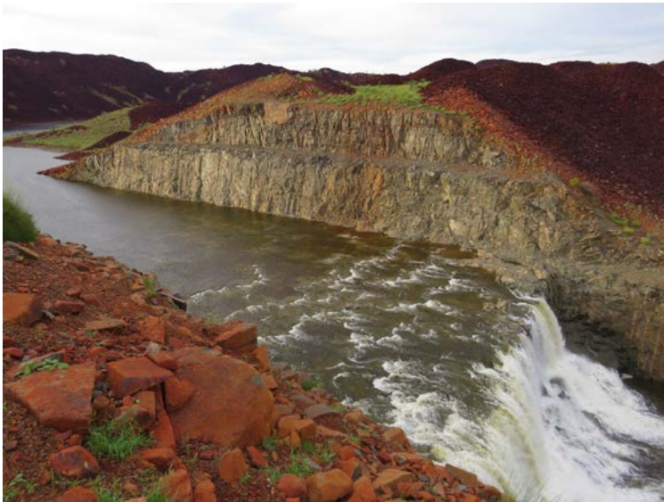
Figure 30: Harding Dam overflowing
