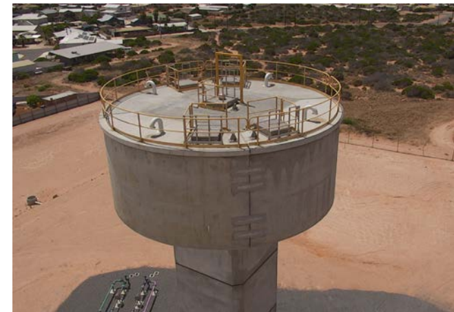
Figure 28: Denham elevated tank
