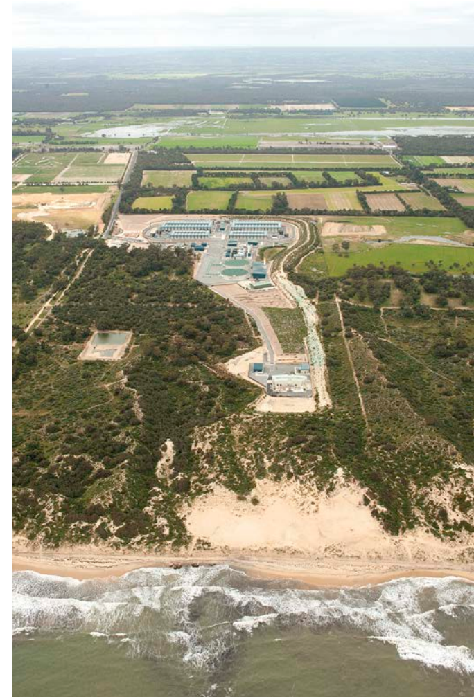
Figure 5: Southern Seawater Desalination Plant (Source: Water Corporation)
