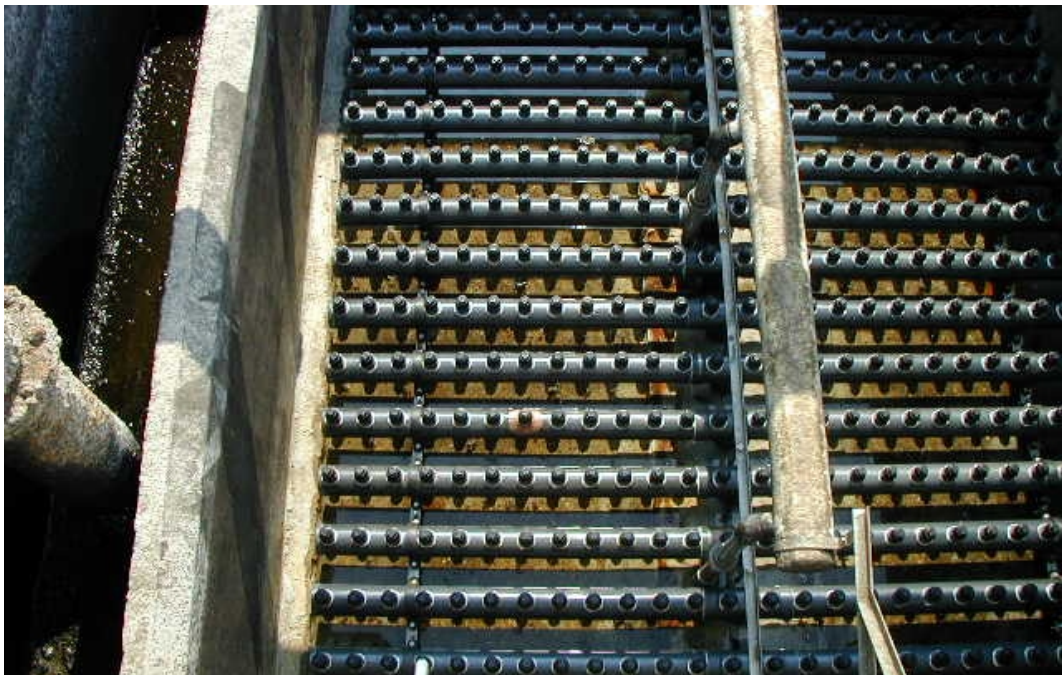
Figure 5.2: Example of a header and lateral floor.
