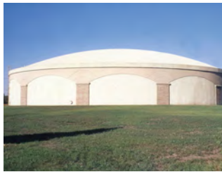
Above Ground Storage Tanks
