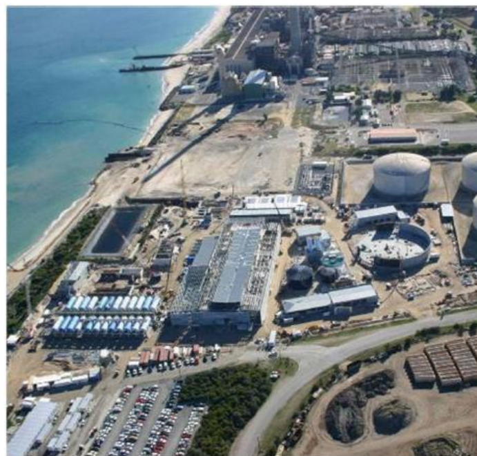
Figure 7-12: Perth SWRO Desalination Plant
