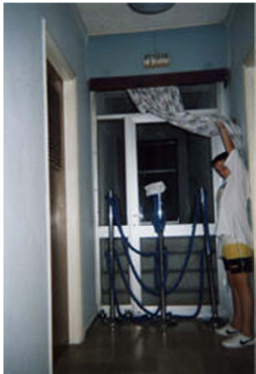
Blocked Fire Exit
