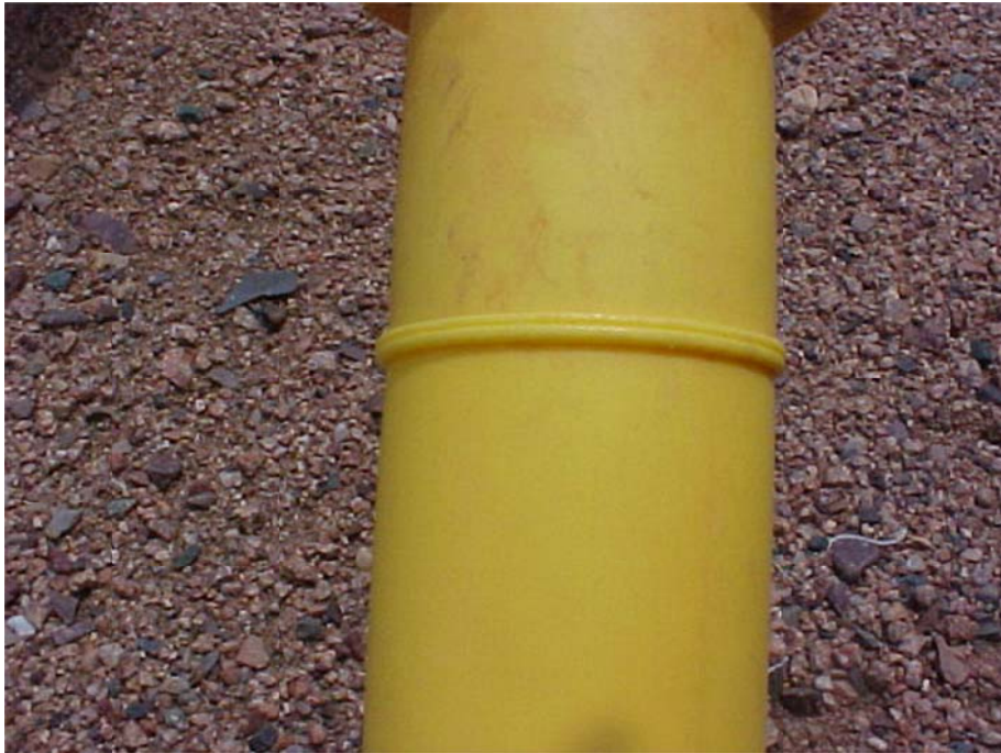
Fusion Butt Joint on plastic pipe.
