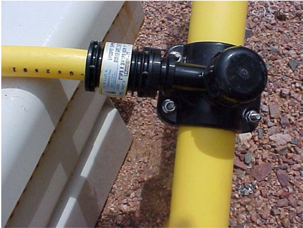
2 x ¾ inch mechanical service tap.
