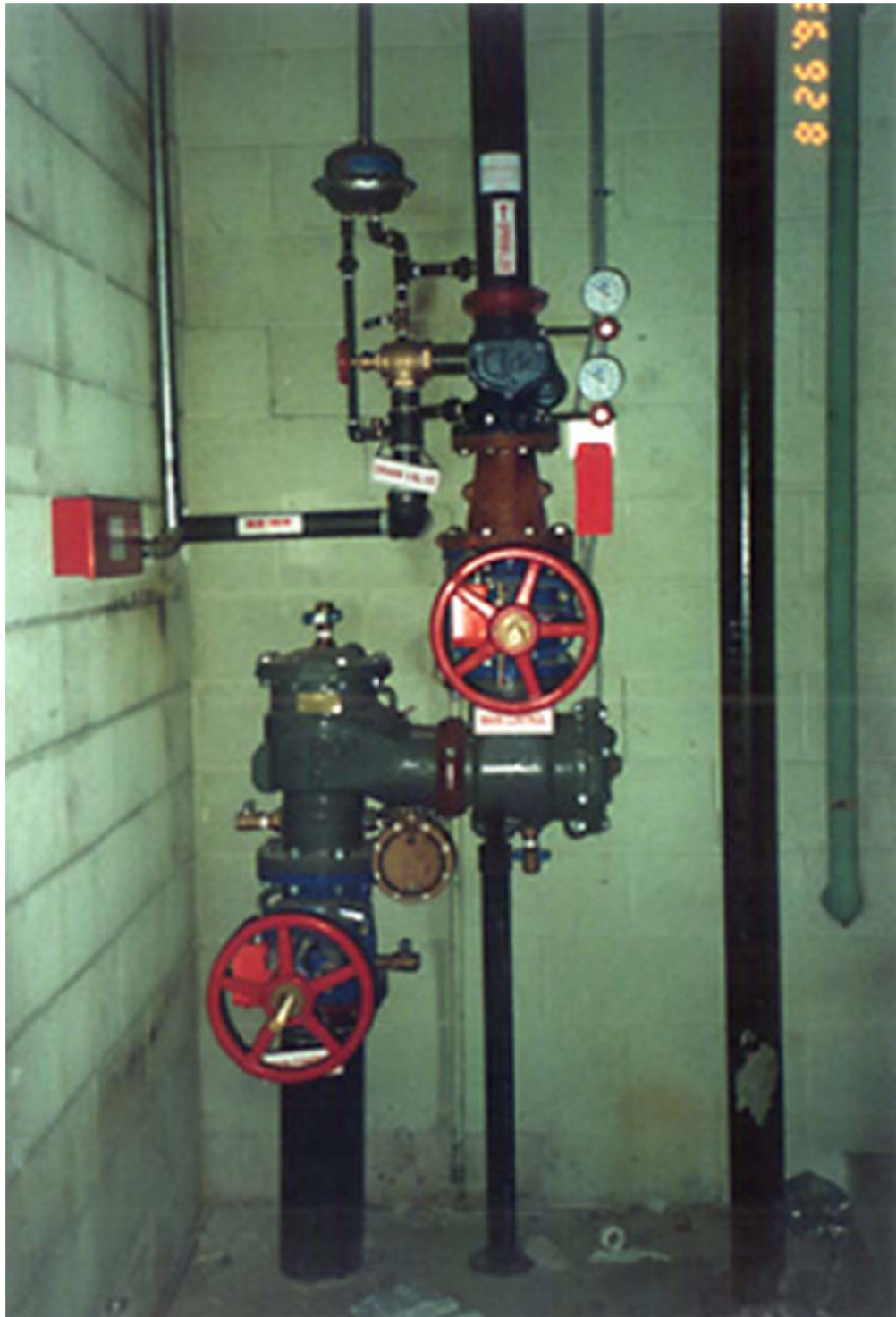
Reduced Pressure Backflow Assembly. A device to prevent contaminants from backflowing into the public water system.
