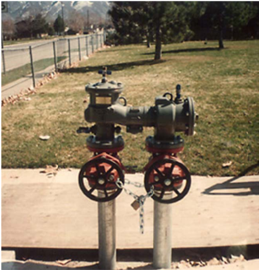
Double Check Backflow Assembly (Notice chain).
