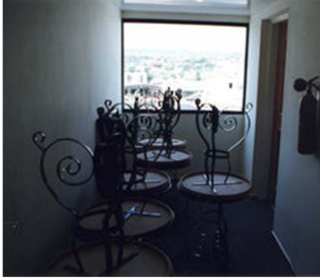
Blocked Fire Exit
