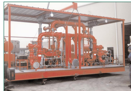
Photo 1. Fire water pump with diesel engine and air start with a nitrogen back-up system
