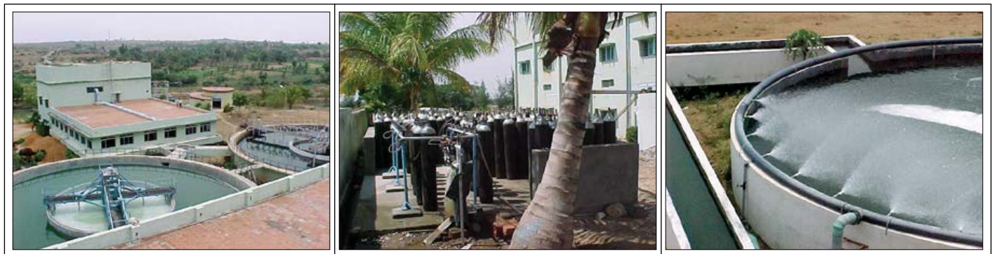
Fig.9. The high pH water in clariflocculators, CO2 cylinder bank and carbonation tank
