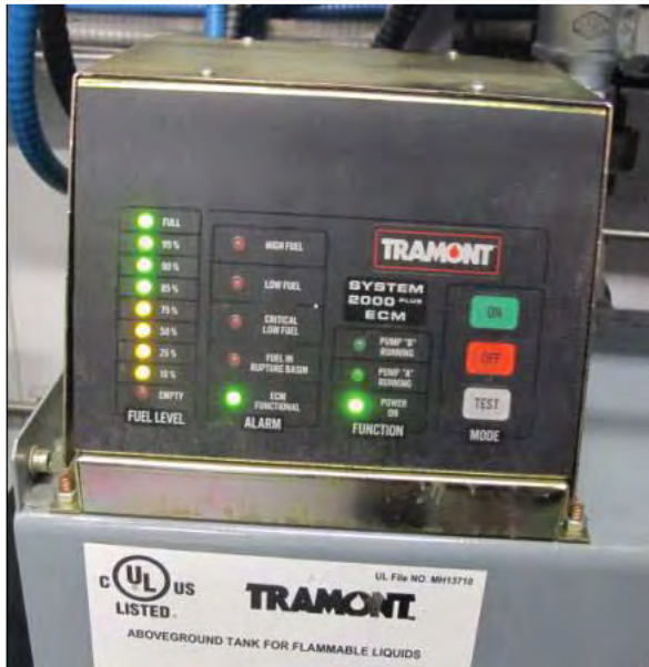
Figure 7. 9: Diesel Day Tank Stop Button
