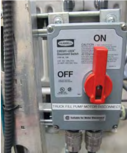
Figure 7. 5: Raw Water Pump Disconnect
