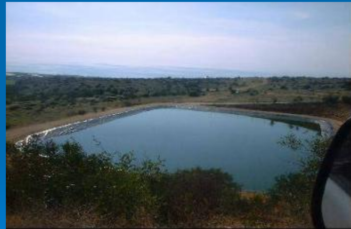
Storage Tank (Secondary treated water)
