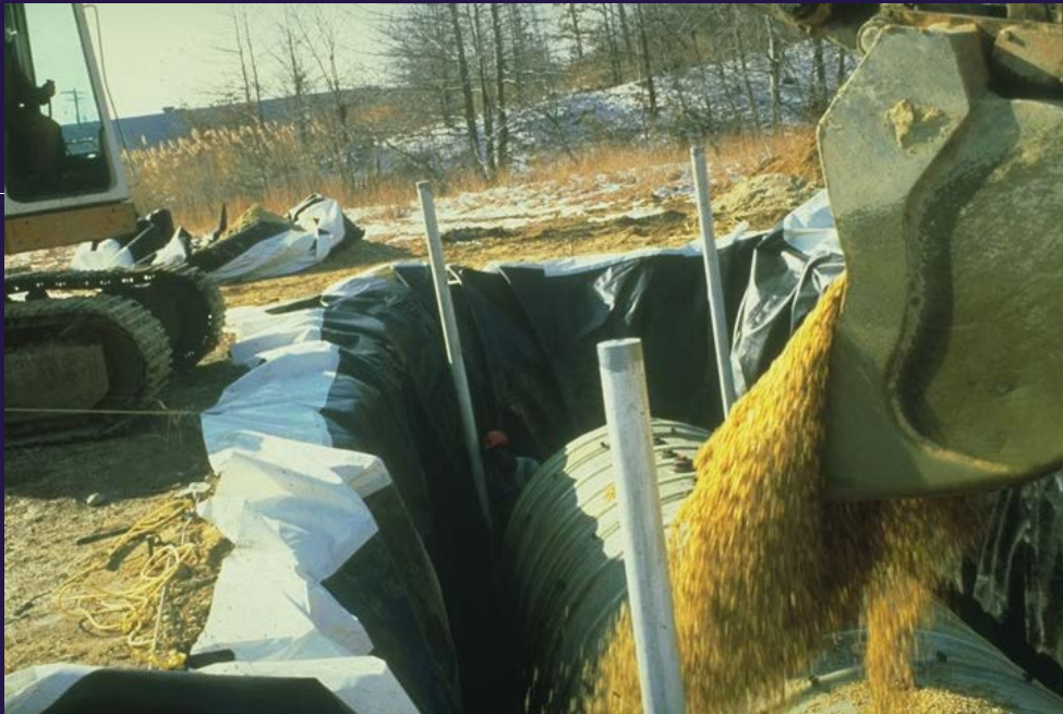
Backfilling a UST installation in a lined pit
