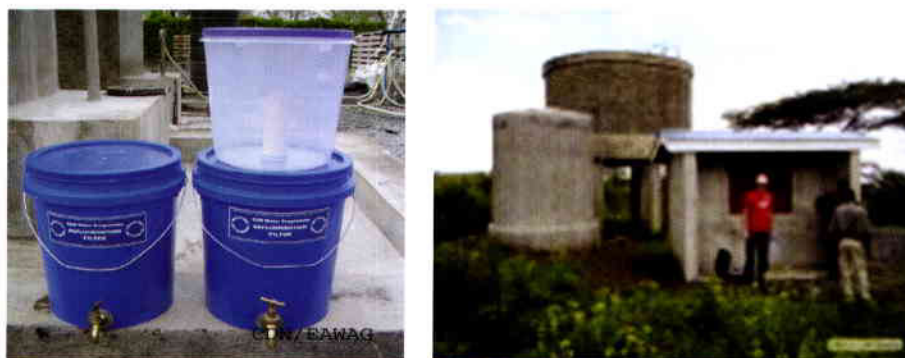
Figure 3.3: Eawag Fluoride Removal by Bone Char
