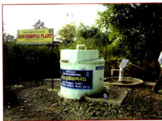
Figure 5.1: NEERI Hand Pump Attachable Iron Removal Plant
