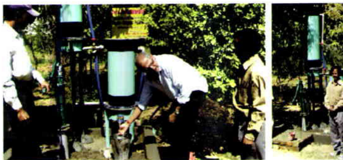
Figure 4.27: Arsenic Removal Plant At Rampur - Maner
