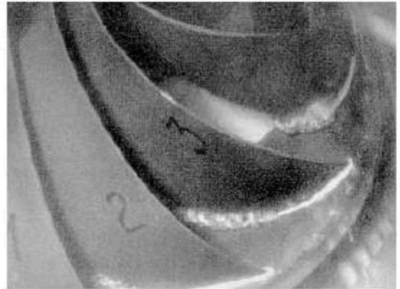
Inlet edge cavitation in Francis turbine
