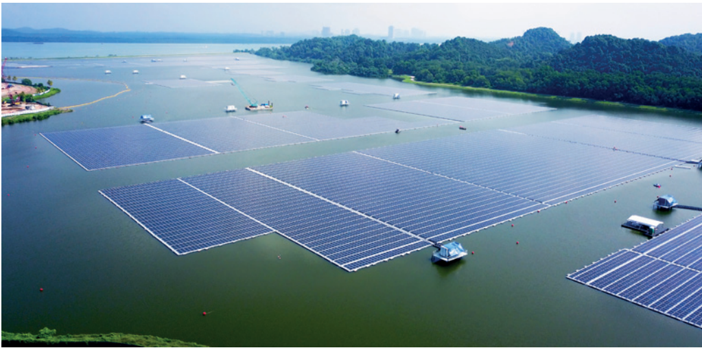
Figure 6. An aerial view of the Tengoh Floating Solar Farm which was launched in July 2021. This solar farm has a peak capacity of 60 megawatts, enough to power 16,000 four-room HDB flats for a year. Photo credit: Sembcorp Industries
