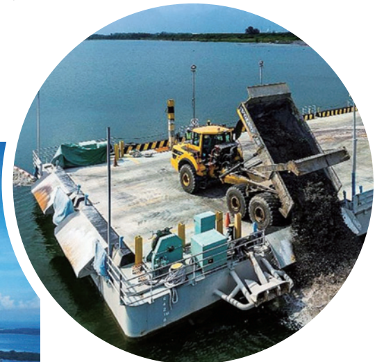
Figure 5. The offshore landfill at Semakau (left image) was created by building a 7km rock bund around Pulau Semakau, Pulau Sakeng and the surrounding waters, to create space where incineration ash generated from waste on the mainland is deposited (top image). This solution has a finite capacity. Photos credit: National Environment Agency
