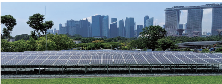
Figure 2. While skyscrapers can be seen in the background, the Marina Barrage PV modules enjoy unblocked access to sunlight due to their unique location at the mouth of the Marina Bay.
