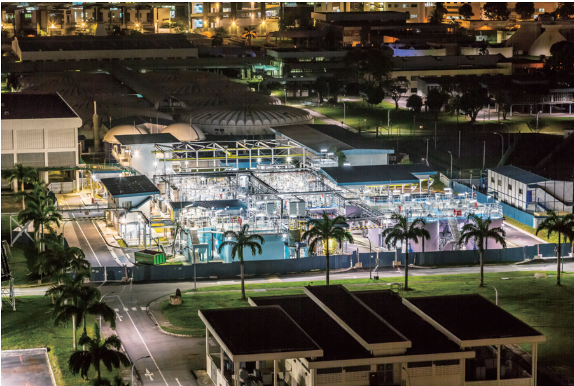
Figure 3. Enhanced primary treatment processes with biosorption were trialled on a smaller scale at a demo plant in Ulu Pandan WRP (left), and found to increase energy recovery while reducing downstream treatment energy requirements before being incorporated into the TWRP's design.
