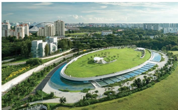
Figure 3. The Keppel Marina East Desalination Plant sits underneath a sprawling green park space where panoramic views of the city skyline can be enjoyed. Photo credit: Keppel
