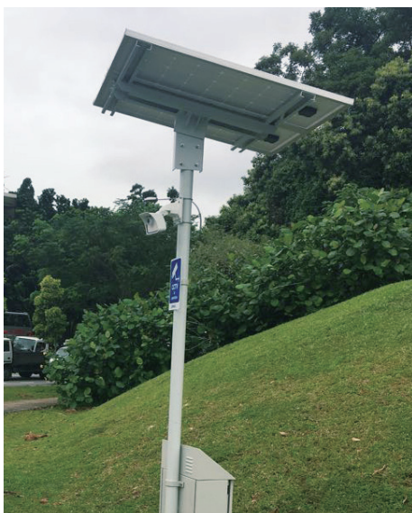
Figure 1. CCTVs are designed to record and monitor scenes. However, by harnessing advanced technologies, they can be also be used as a rain gauge.
