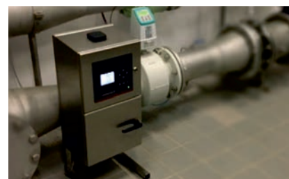
Figure 2: Example of BACMON bacteria sensor installation along distribution pipe
