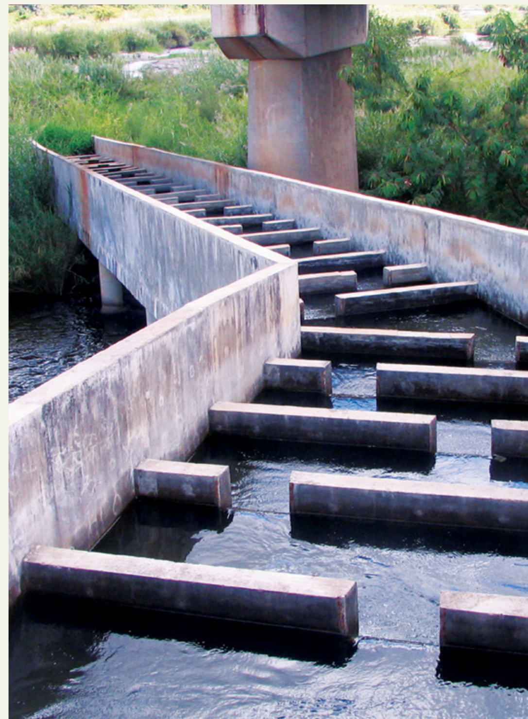
Fish ladder in the Inkomati catchment, to facilitate fish migration through the river system. “With the addition of our new flood forecasting system we now have a catchment-wide system where we’re basing our decisions on information available, in real-time, at our fingertips, and we have far better knowledge of what’s going on in the catchment, and how to respond,” says Brian Jackson, IUCMA’s executive manager for water resources planning.
