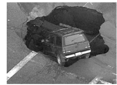
Sink hole caused by 8-in main break
