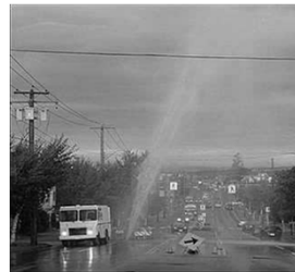
Sink hole caused by 8-in main break
