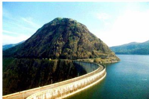
Fig.1.4. Reservoir. (Idukki Arch dam -Kerala, India).
