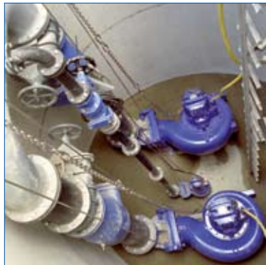
Fig. 2.12b: Guide wire arrangement
