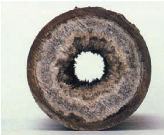
Photo 10.8 Scale in the piping under no chemical treatment
