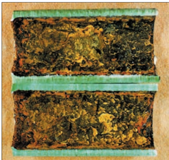
The whole surface of carbon steel is covered with the corrosion products.
