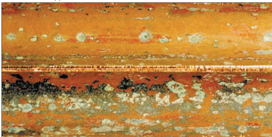
The average corrosion rate of copper and copper alloys is generally low in cooling water systems, but they are often attacked by local corrosion with the green rust composed of basic cupric sulfate and so on under no chemical treatment.
