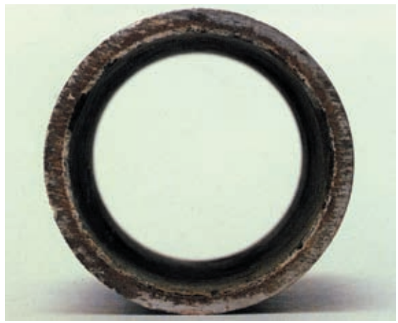
Photo 10.9 Clean piping treated with a scale inhibitor
