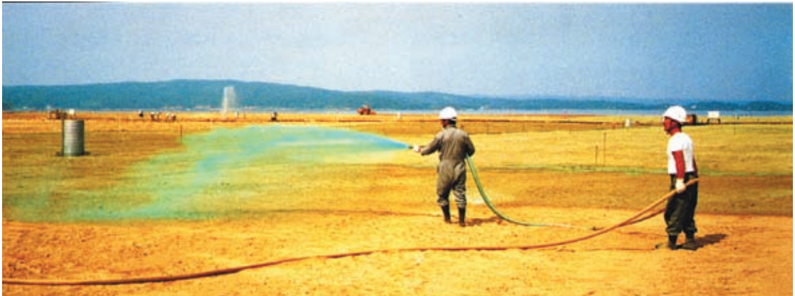
Photo 10.20 Sprinkling of a dust blow-away preventive solution on a reclaimed land
