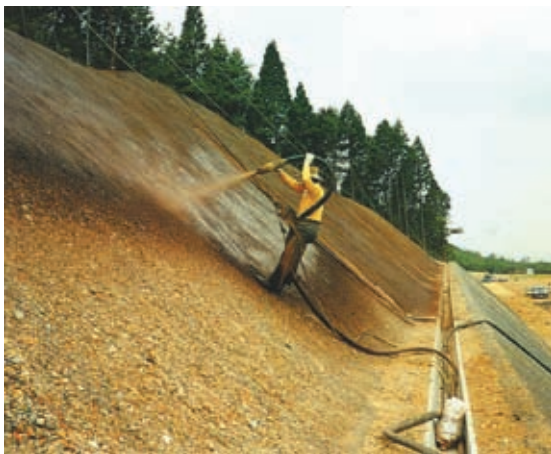
Photo 10.17 Sprinkling of the mixture of a dust blow-away preventive and grass seeds by a pump pressure
