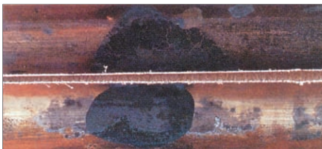
Photo 5.9 Non-uniform oxide film on the copper tube inside of an air handling unit before the use
