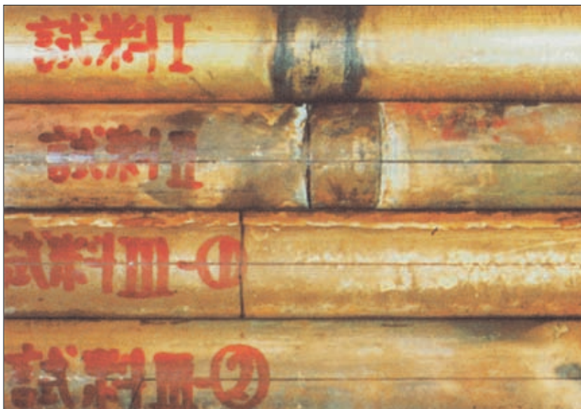
Photo 2.9 Corrosion of steam condenser tubes (aluminum brass)
