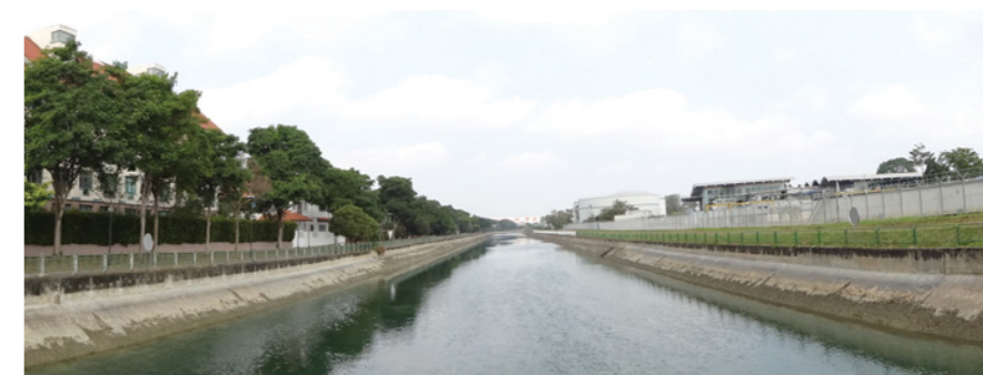
Existing condition of the stretch of Bedok Canal to be upgraded.
