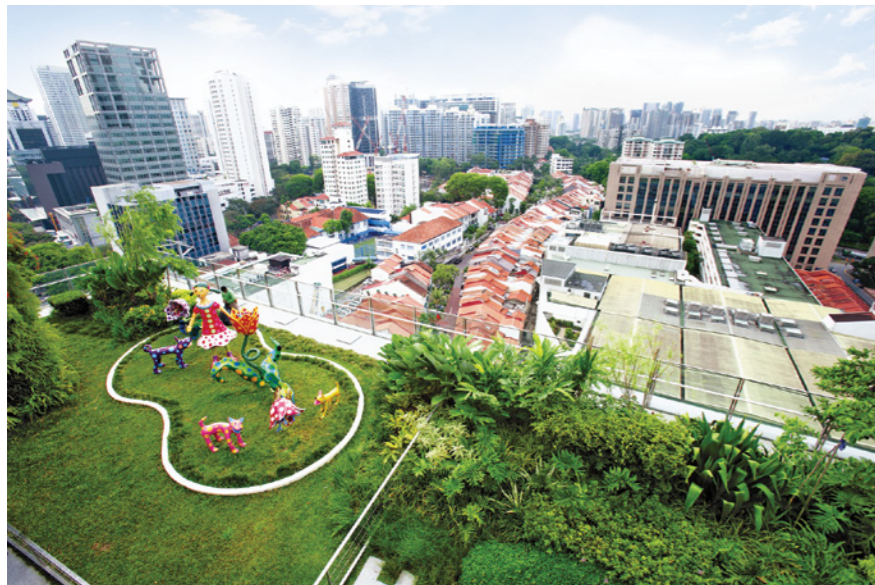
A landscaped green roof and rooftop garden on top of Orchard Central Mall: The rooftop vegetation captures rainwater, allowing evaporation and evapotranspiration processes to take place and reducing the amount of runoff entering downstream drainage systems.
