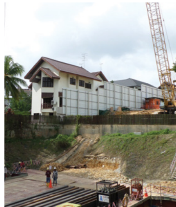
Upgrading works in progress
