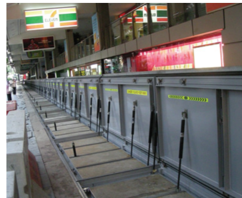
Minimum crest levels at entrances to basements can be achieved with, for example, ramps (left) or automatic flip-up flood barriers (right).
