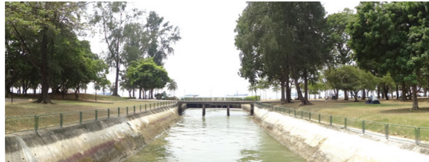
Existing condition of the stretch of Siglap Canal to be upgraded from 2014 to 2016.
