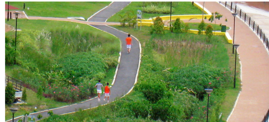
A bioretention basin (or rain garden) at Balam Estate: Runoff is first filtered through densely planted surface vegetation and then through an engineered filter media layer. The filtered runoff is then collected via a perforated pipe at the bottom drainage layer and discharged to the nearby canal.
