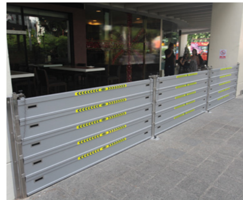
Steps and ramps are some of the ways to achieve the minimum platform levels for developments (left). Alternatively, flood barriers can be manually installed when needed (right).
