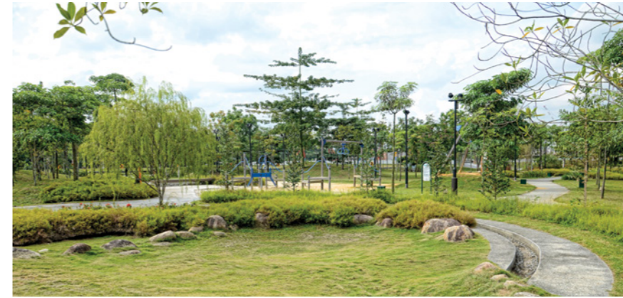
A dry pond at Greenwood Sanctuary: During rain events, runoff from the surrounding area flows to the dry pond and infiltrates through the filter media to underground percolation tanks. During dry weather, the lawn area in the dry pond can be used for recreational activities.
