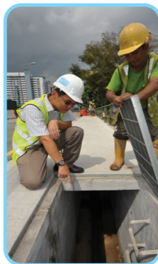
Inspecting the condition of our drains
