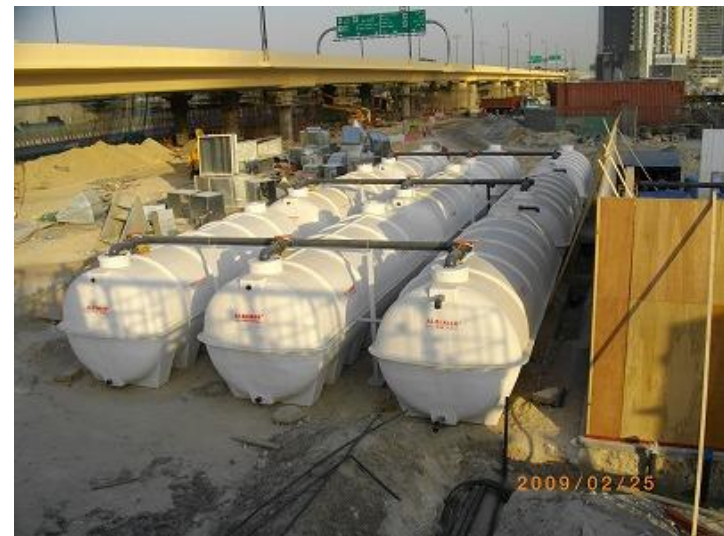
TSE WATER TANK
