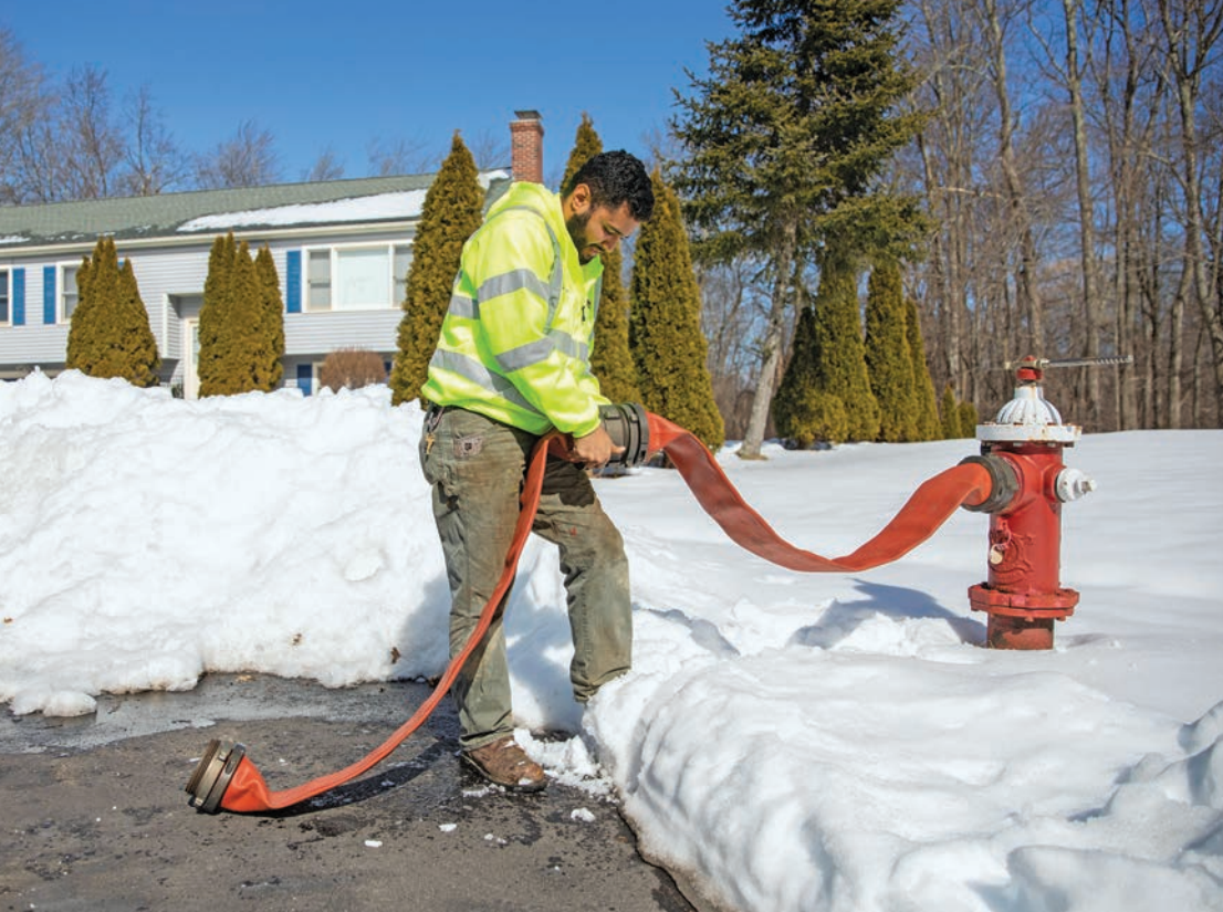
Jonathan Gonzalez-Rosario attaches a hose to a fire hydrant before flushing a segment of the water system.
