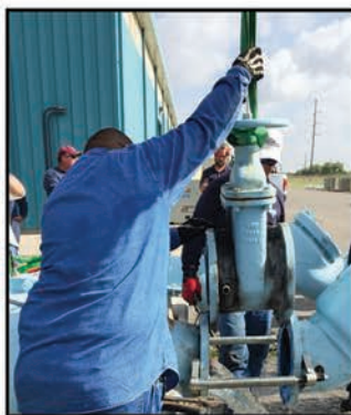
Spread outside flanges & remove old valve
