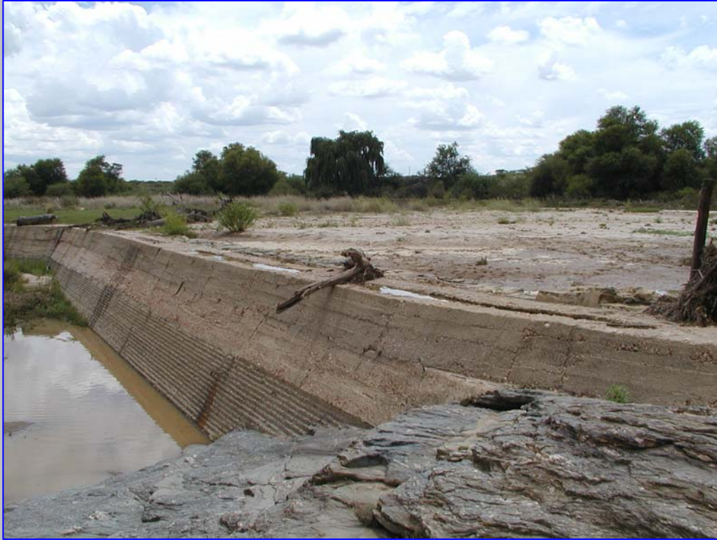
1. Sand dam after first flood
