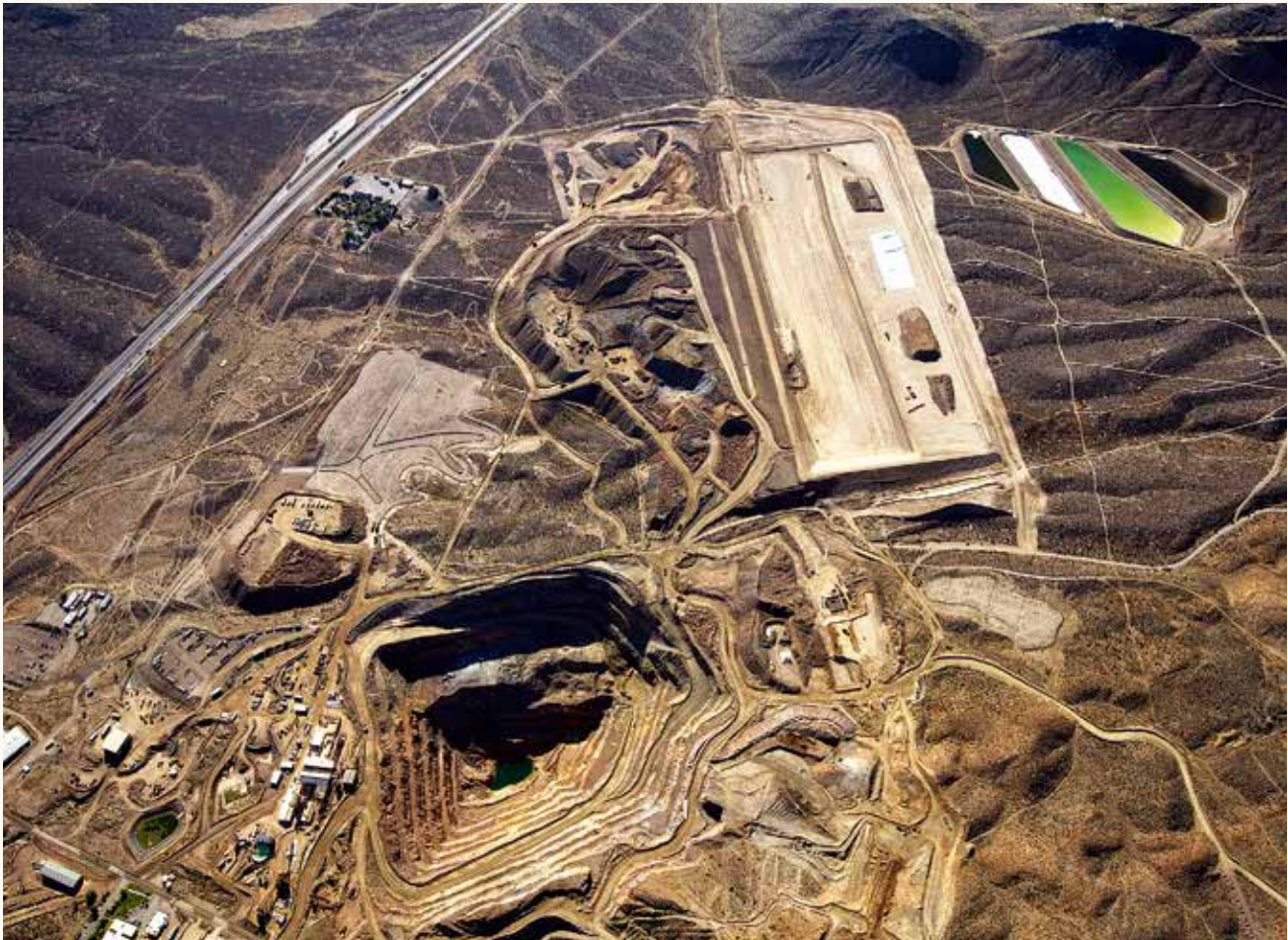
REE open pit mine located in California, USA. Most REE-mining is carried out in similarly arid environments in China.
