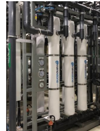
Grind WW (retrofit)
